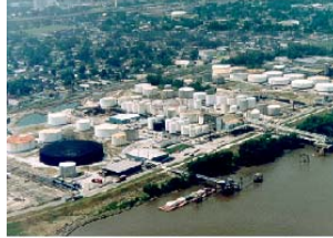
Bulk Fuel Storage
